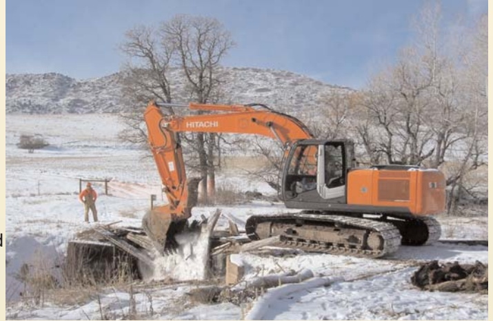
Breaking ground for the entry road leading into Hildebrand Ranch Park.
